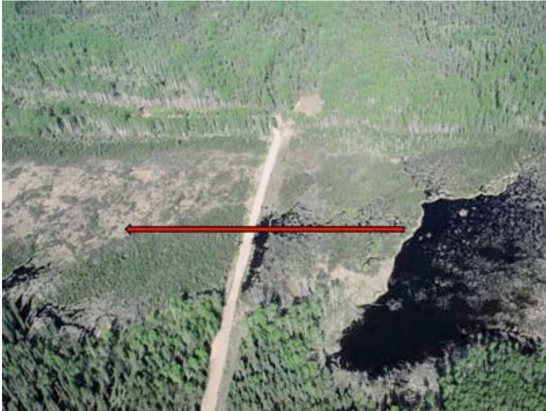
Road blocking water flow through boreal wetland
