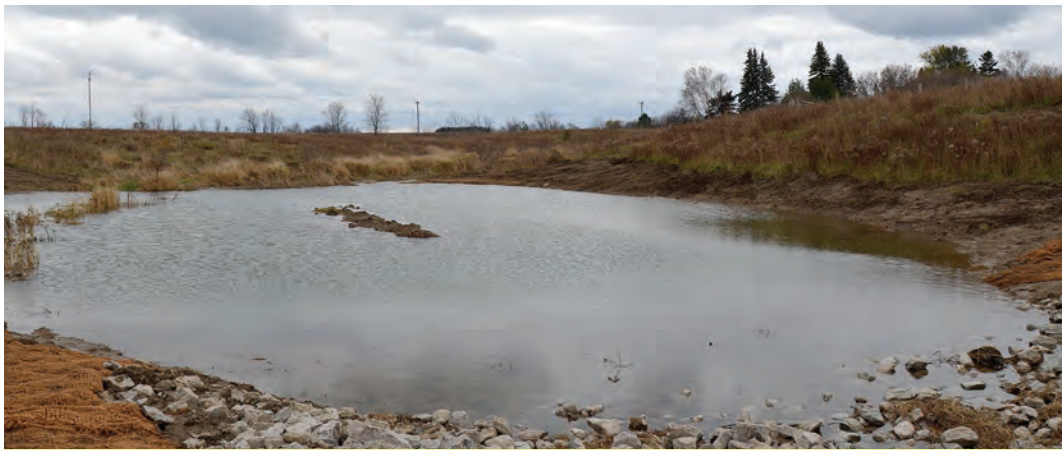
Above: New DUC wetland restoration project in Tiny Township
