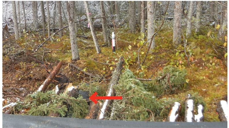
Figure 2. View of a well next to the road. The crossing structure being monitored is a log-corduroy crossing with a plastic culvert (red arrow points to culvert inlet).
